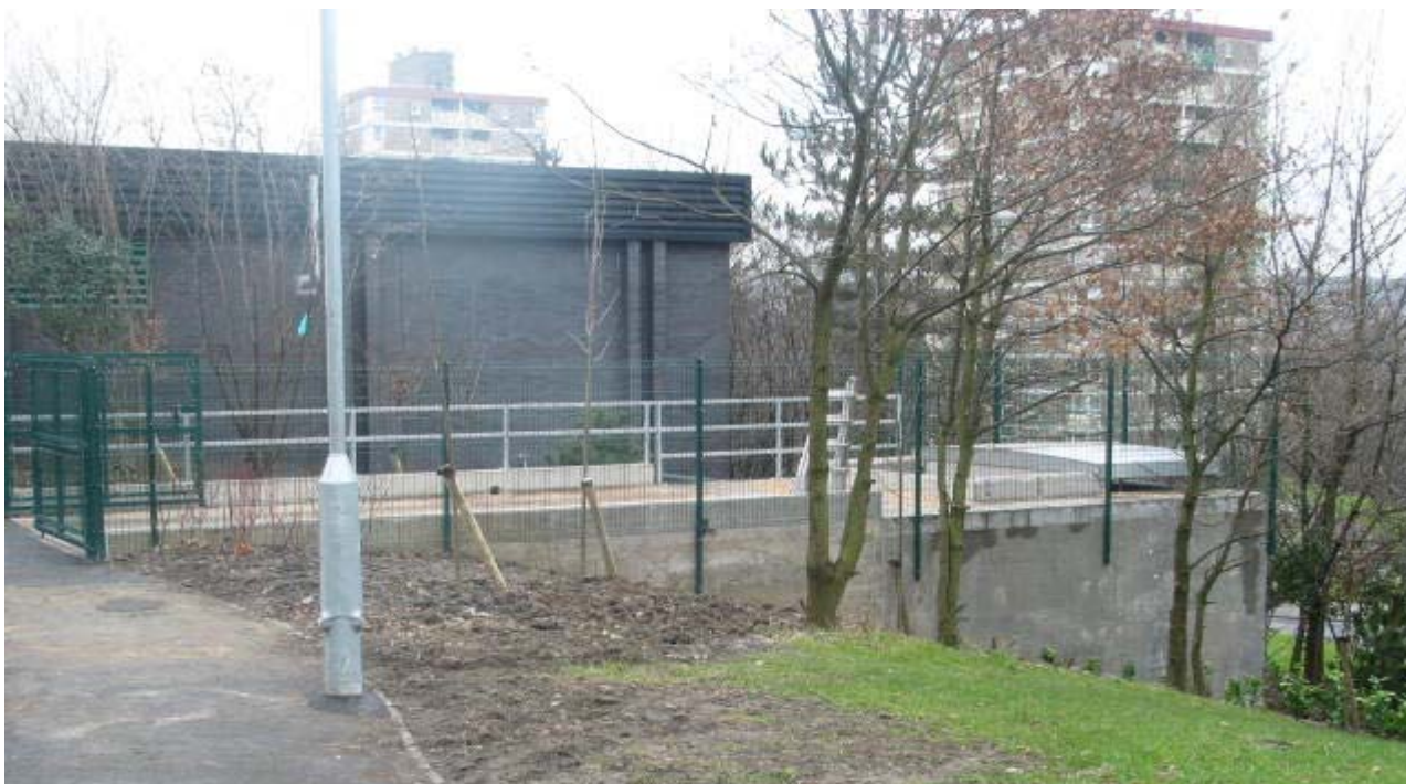
Boiler room (behind) & fuel reception bunker
