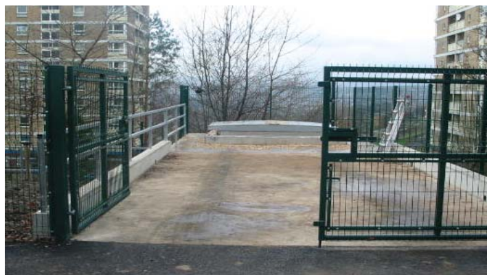
Fuel reception bunker
